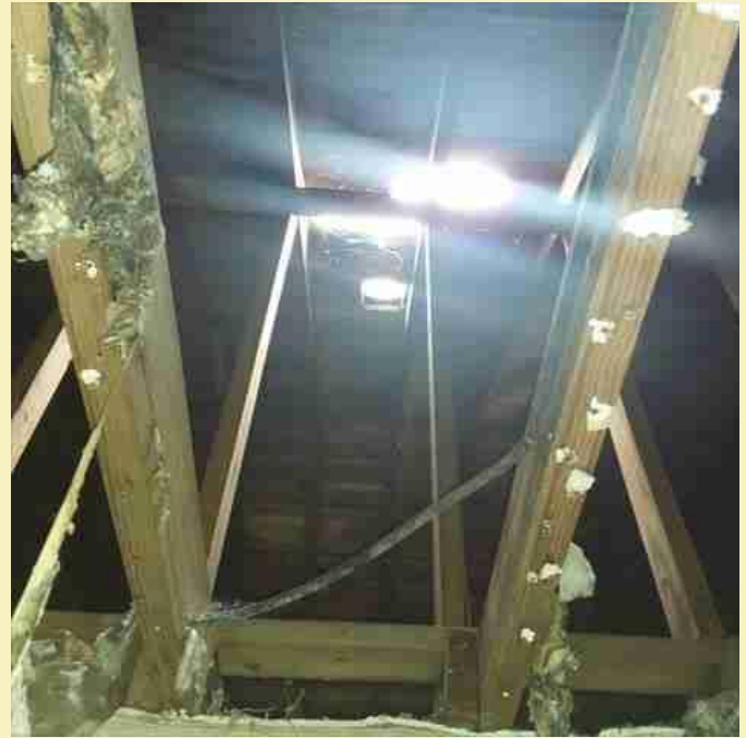
Here is the roof over what I think was my bedroom
